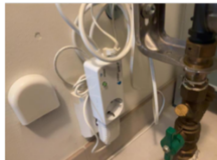
Montert vannstopper system
